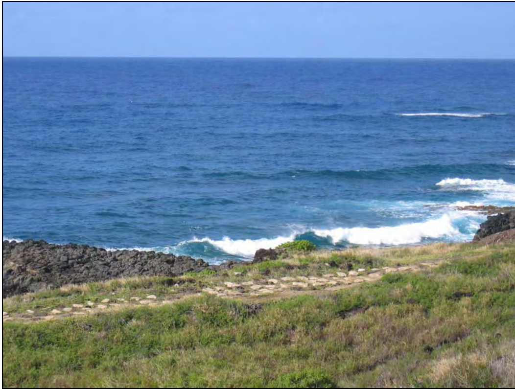
Fig. 25: Limestone Slab Pavement on Railway Bed near Southern Extent of Project Area (Facing Southwest).
