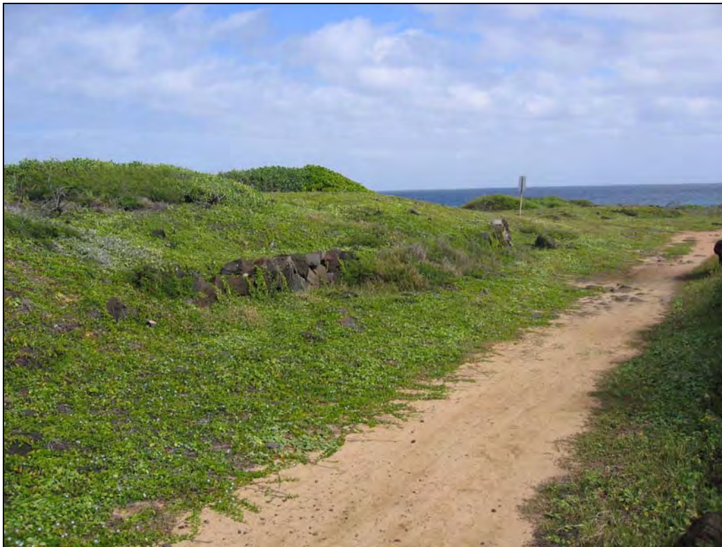
Fig. 28: Rock Retaining Wall along Makai Edge of Railway Bed near Northern Bend in the Alignment (Facing North). Note use of angular stones.
