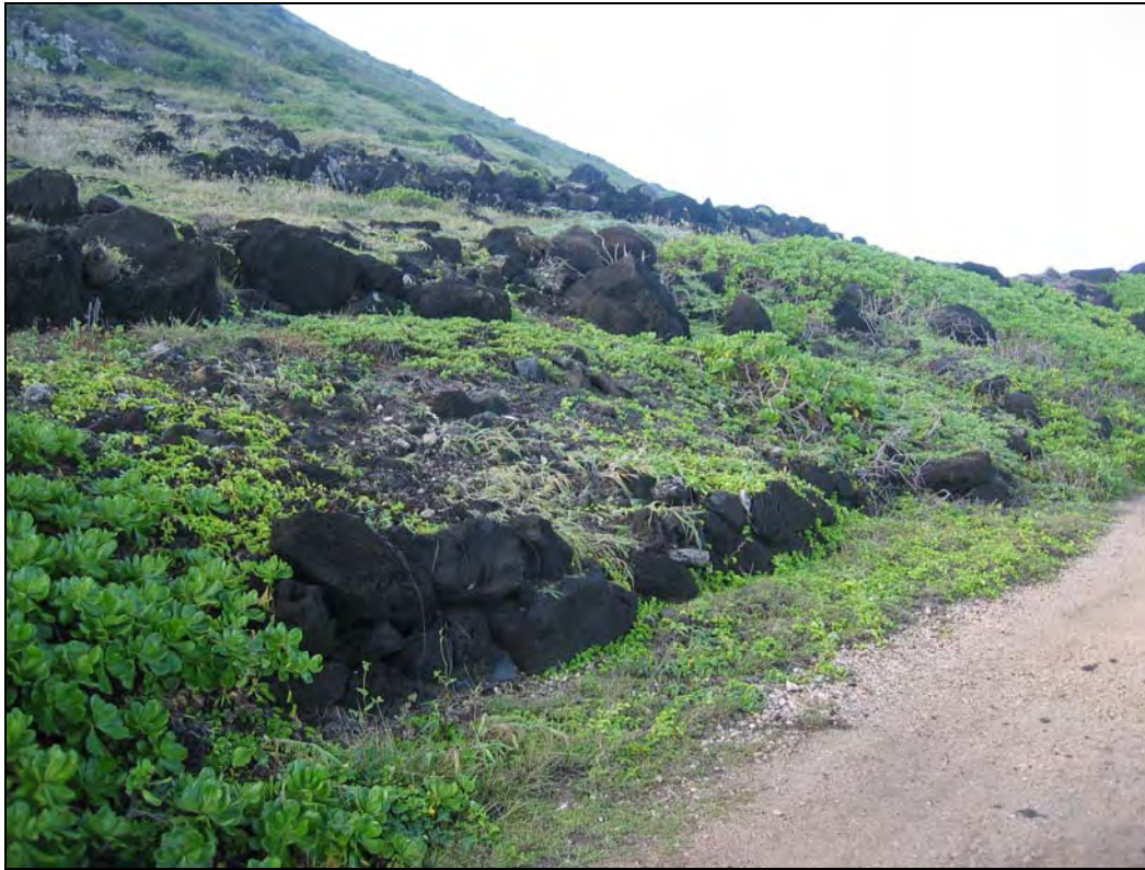
Fig. 27: Rock Retaining Wall along Edge of Railway Alignment near Northeastern Extent of the Project Area (Facing Southeast).
