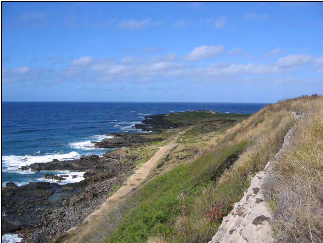
Fig. 34: Gunite-Coated Retaining Wall along Cut and Fill Gravel Road Beyond BCN-409 Southern Tunnel (Facing Northwest).
