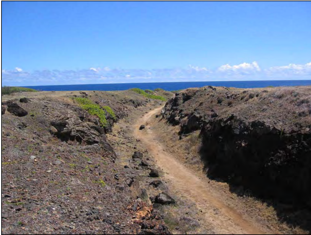
Fig. 23: Railway Bed Cut at Major Bend in the Right-of-Way (Facing North).
