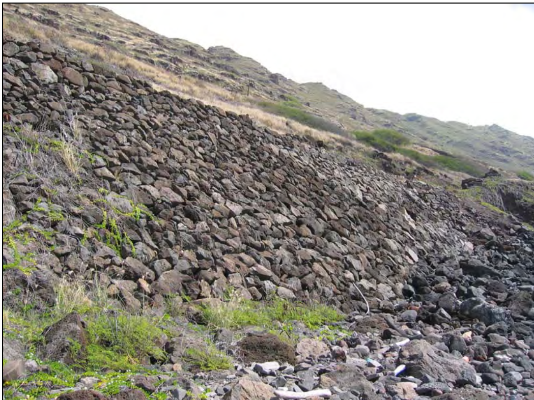
Fig. 22: Close-Up of Rock Retaining Wall for Railway Bed (Facing Southeast).
