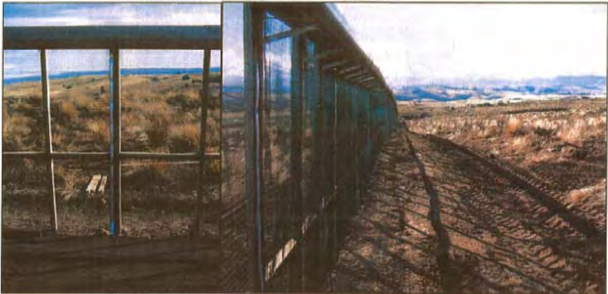
Figure 5. Front and side views of predator-proof fence on rocky terrain in New Zealand.
