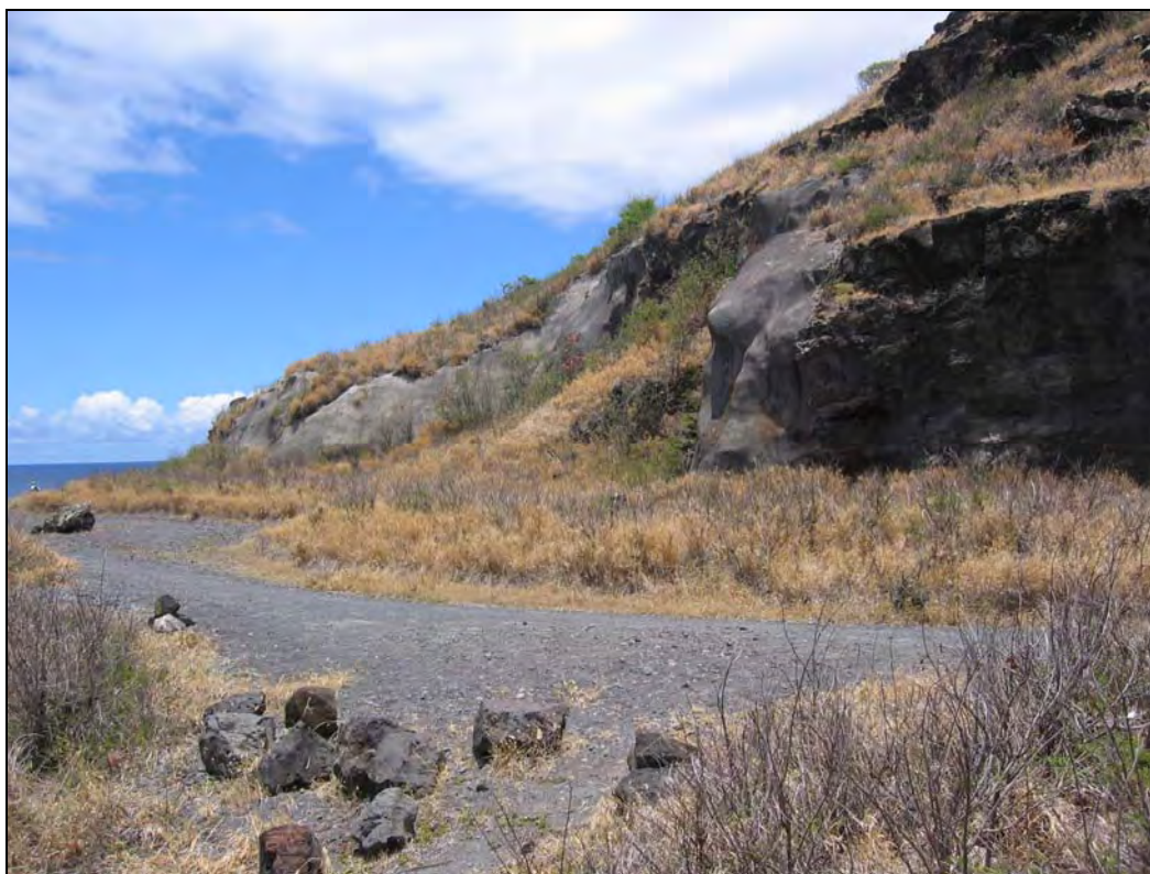
Fig. 32: Sealed Entrance to BCN-409 Northern Tunnel (Facing Northeast). Note Ridge Cuts Stabilized with Pressure-Sprayed Gunite.
