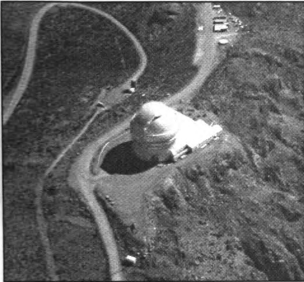
FIGURE 2-20. AERIAL VIEW OF GEMINI SOUTH TELESCOPE
