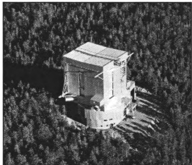
FIGURE 2-28. AERIAL VIEW OF THE LBT ENCLOSURE
