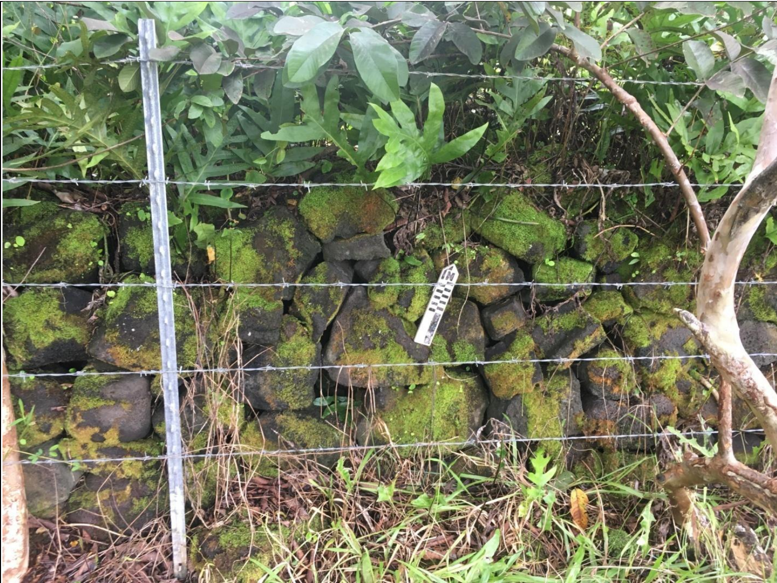
Figure 31: Photograph of Site 31185 Middle Portion of Wall Looking Northwest.
