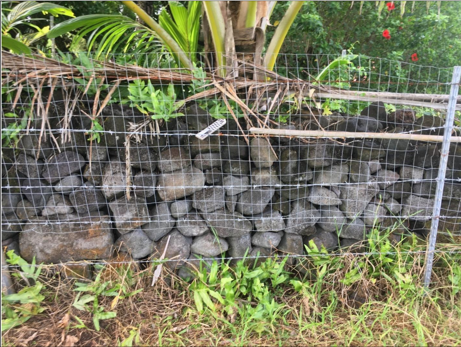
Figure 30: Photograph of Site 31185 Southwest Portion of Wall Looking Northwest.
