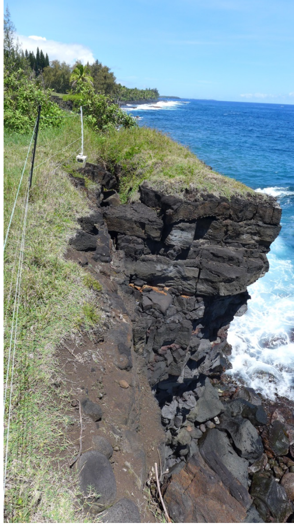
Photo 10 Large pāhoehoe block liable to failure, view to the northwest (noted in Figure 9).
