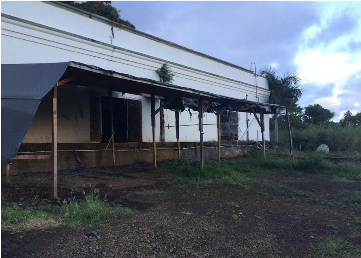
Figure 24. Exterior view of HPCo Warehouse "B," side (northeast) facade, camera facing north (2014). Courtesy Scientific Consultant Services, Inc. (SCS)
