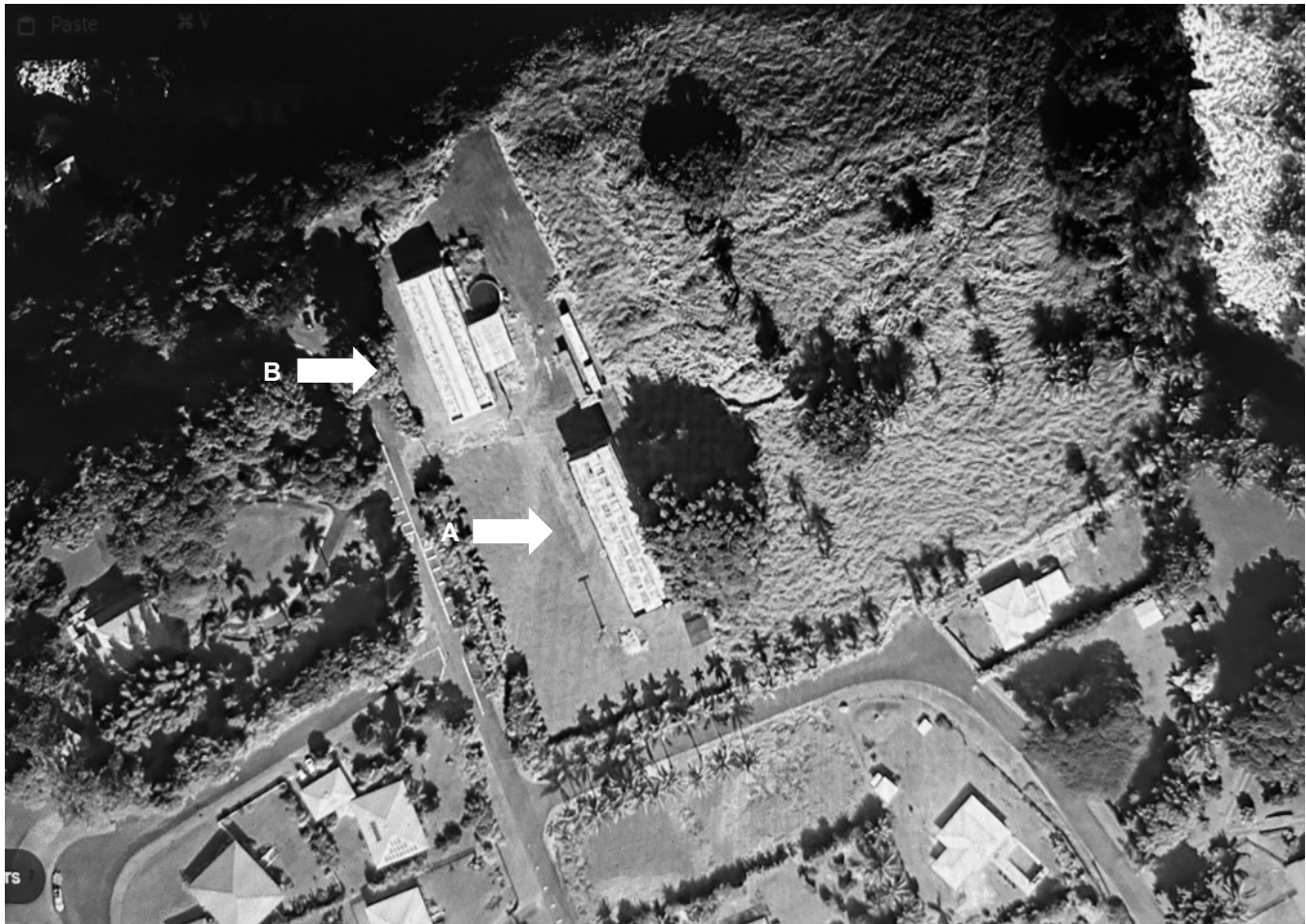
Figure 13. Aerial view of the former HPCo site showing HPCo Warehouse "A" (arrow A) and HPCo Warehouse "B" (arrow B). Courtesy Google Earth (2013).
