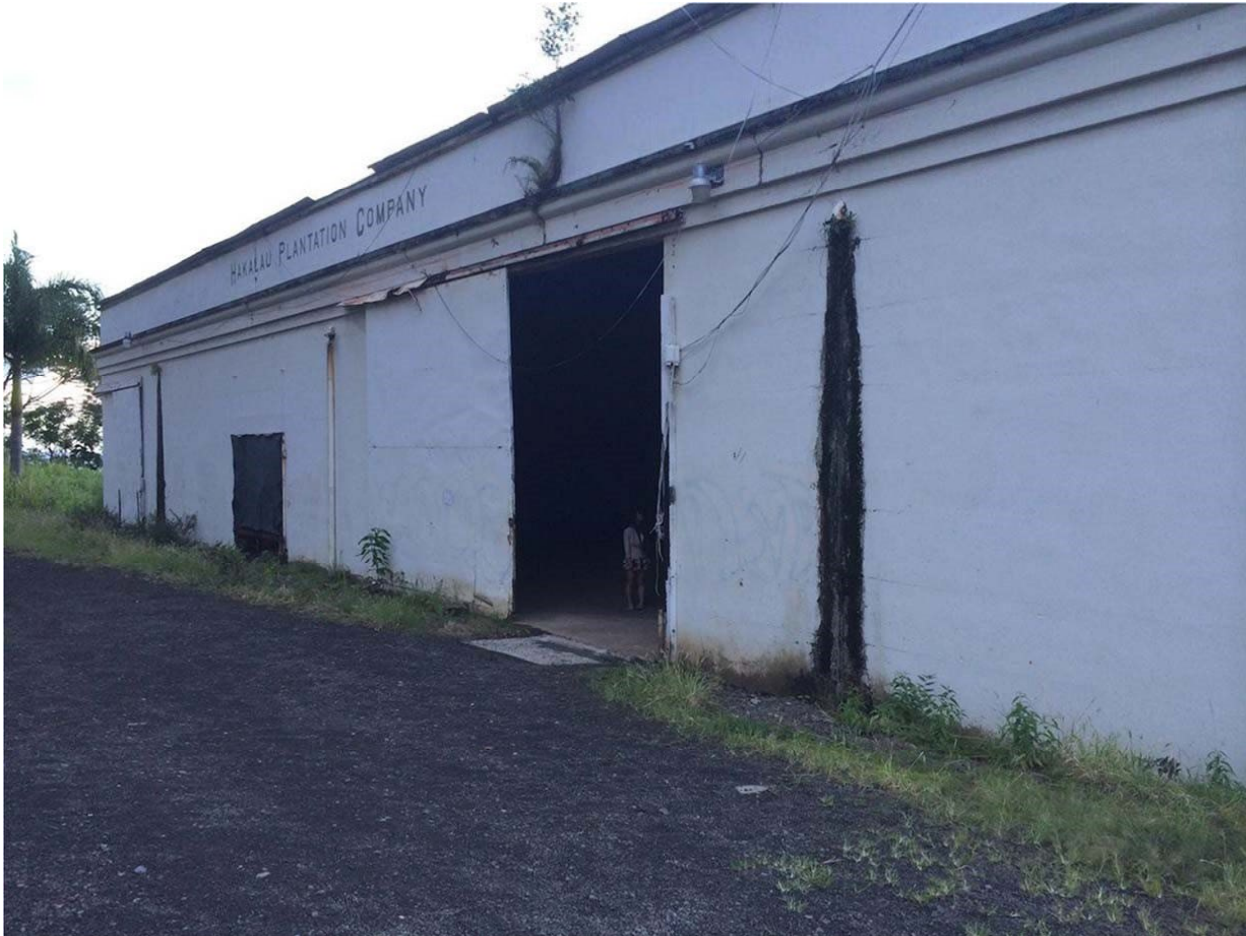
Figure 23. Exterior view of HPCo Warehouse "B," side (southwest) facade, camera facing northeast (2014). Courtesy Scientific Consultant Services, Inc. (SCS)
