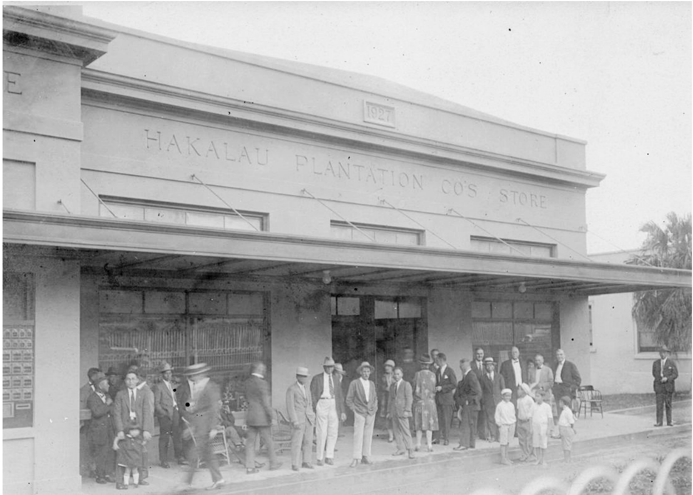
Figure 5. Opening Day at the new Hakalau Plantation Co. (HPCo) Store, January 27, 1928. Photo Courtesy of the Waichi Ouye Collection and Susan Forbes.
