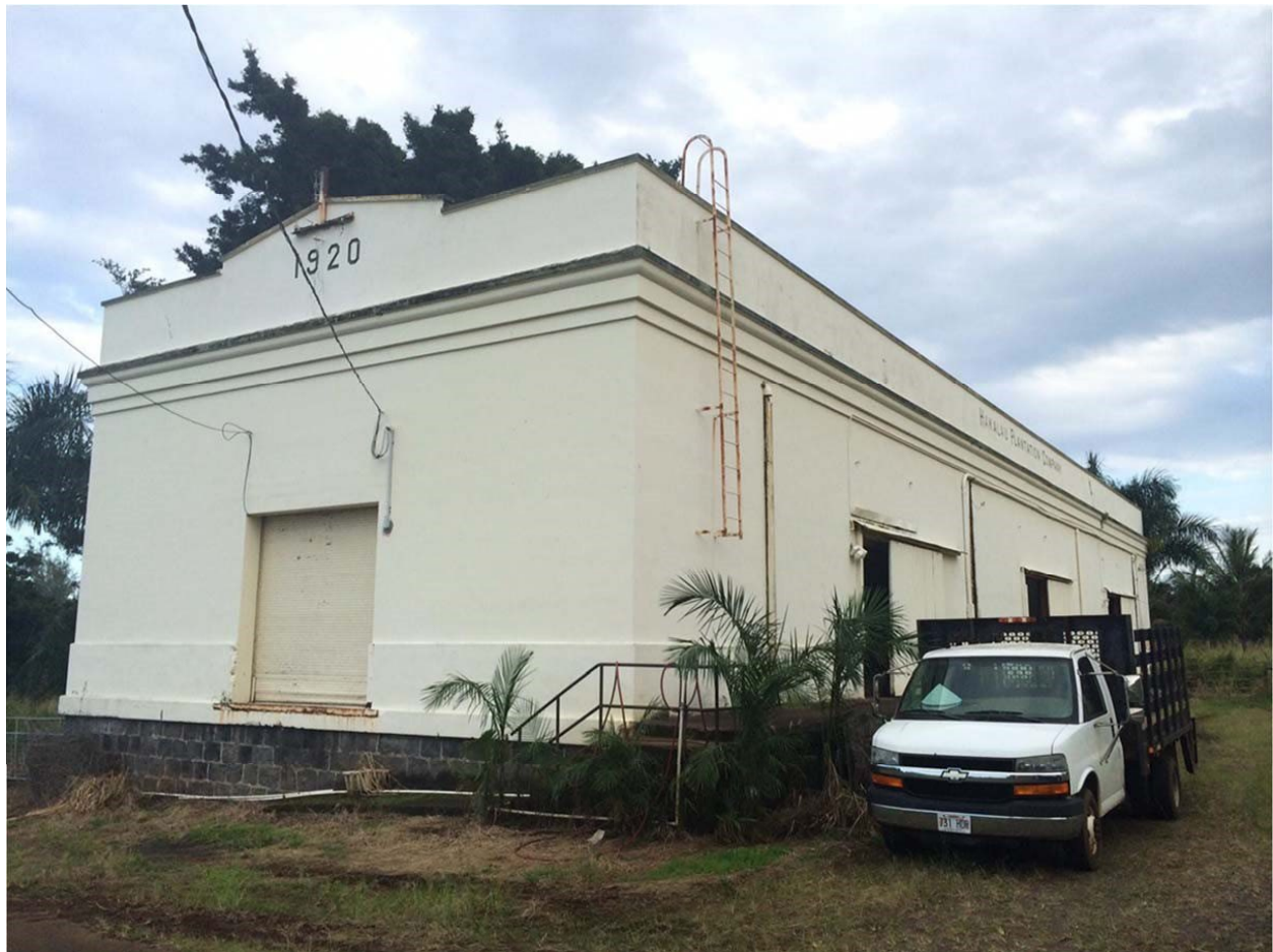
Figure 15. Exterior view of HPCo Warehouse "A," front (northwest) and side (southwest) facades, camera facing southeast (2014). Courtesy Scientific Consultant Services, Inc. (SCS)
