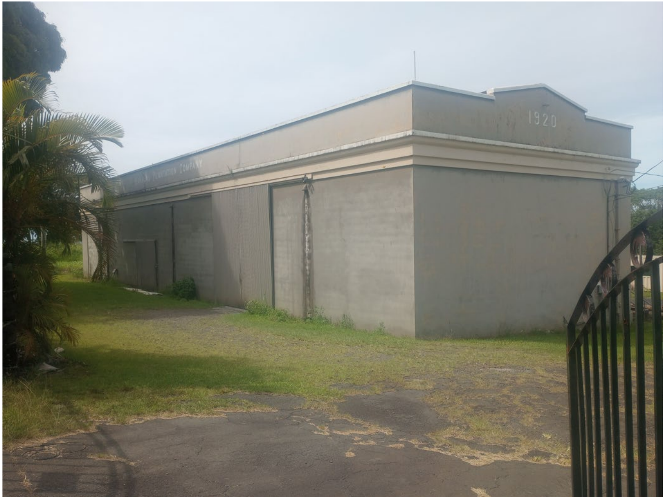
Photo 15 (HI_Hakalau_HPCoWarehouseB_15) HPCo Warehouse "B," oblique view of rear (southeast) and side (southwest) facades, camera facing northeast (2025)
