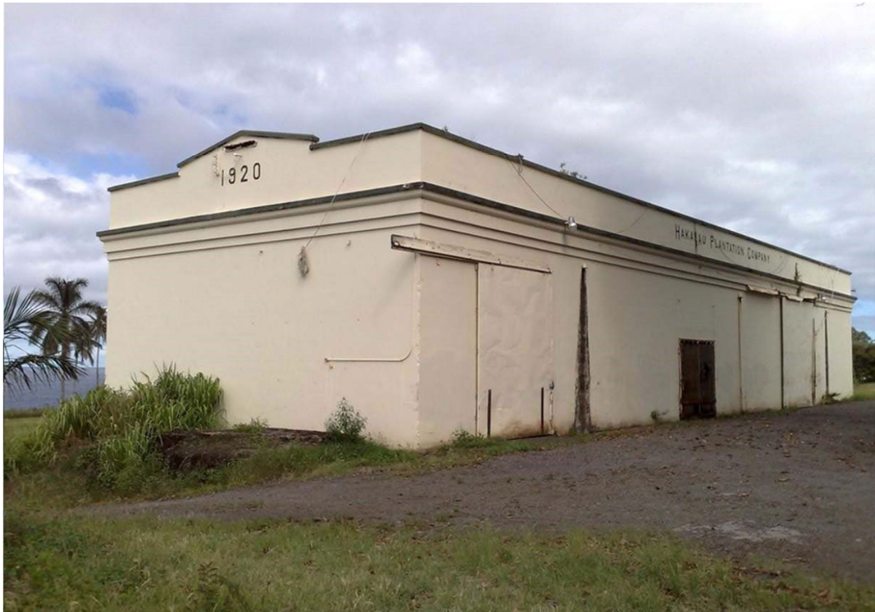
Figure 22. Exterior view of HPCo Warehouse "B," front (northwest) and side (southwest) facades, camera facing southeast (2014). Courtesy Scientific Consultant Services, Inc. (SCS)
