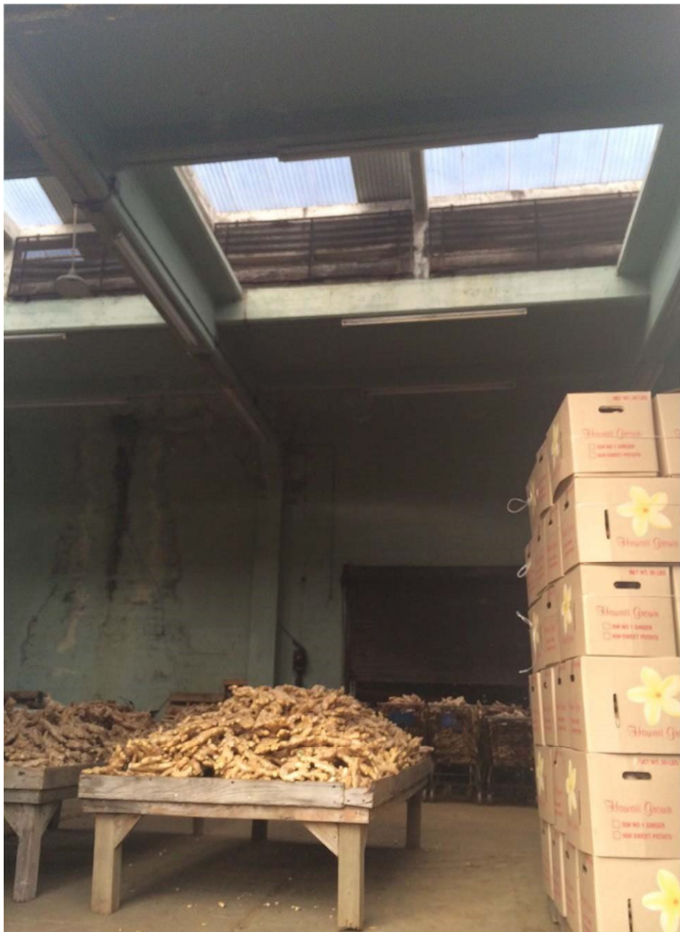
Figure 20. Oblique interior view of HPCo Warehouse "A" roof framing and monitor), camera facing northeast (2014). Courtesy Scientific Consultant Services, Inc. (SCS)
