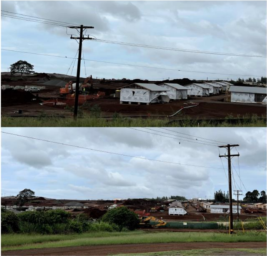
Hōkūau Residential Development under construction
