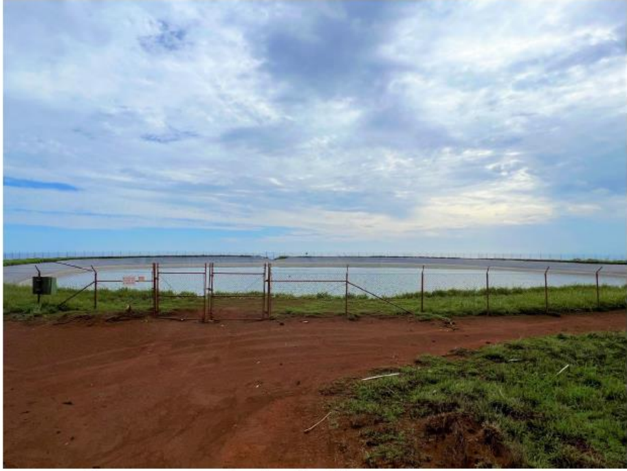
R-1 Water Reclamation Reservoir on the edge of the Pālāwai Basin
