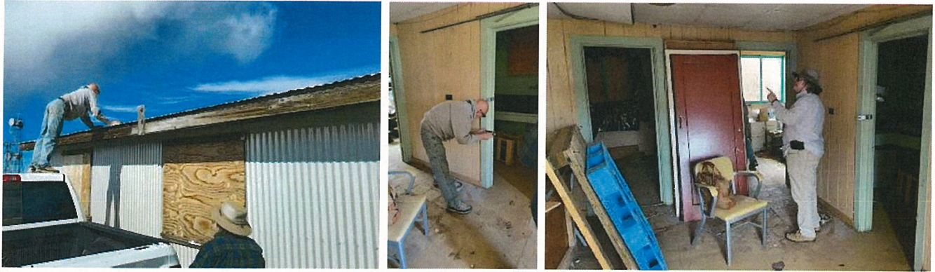
Figure 1. Work in progress at the former Chicago building
