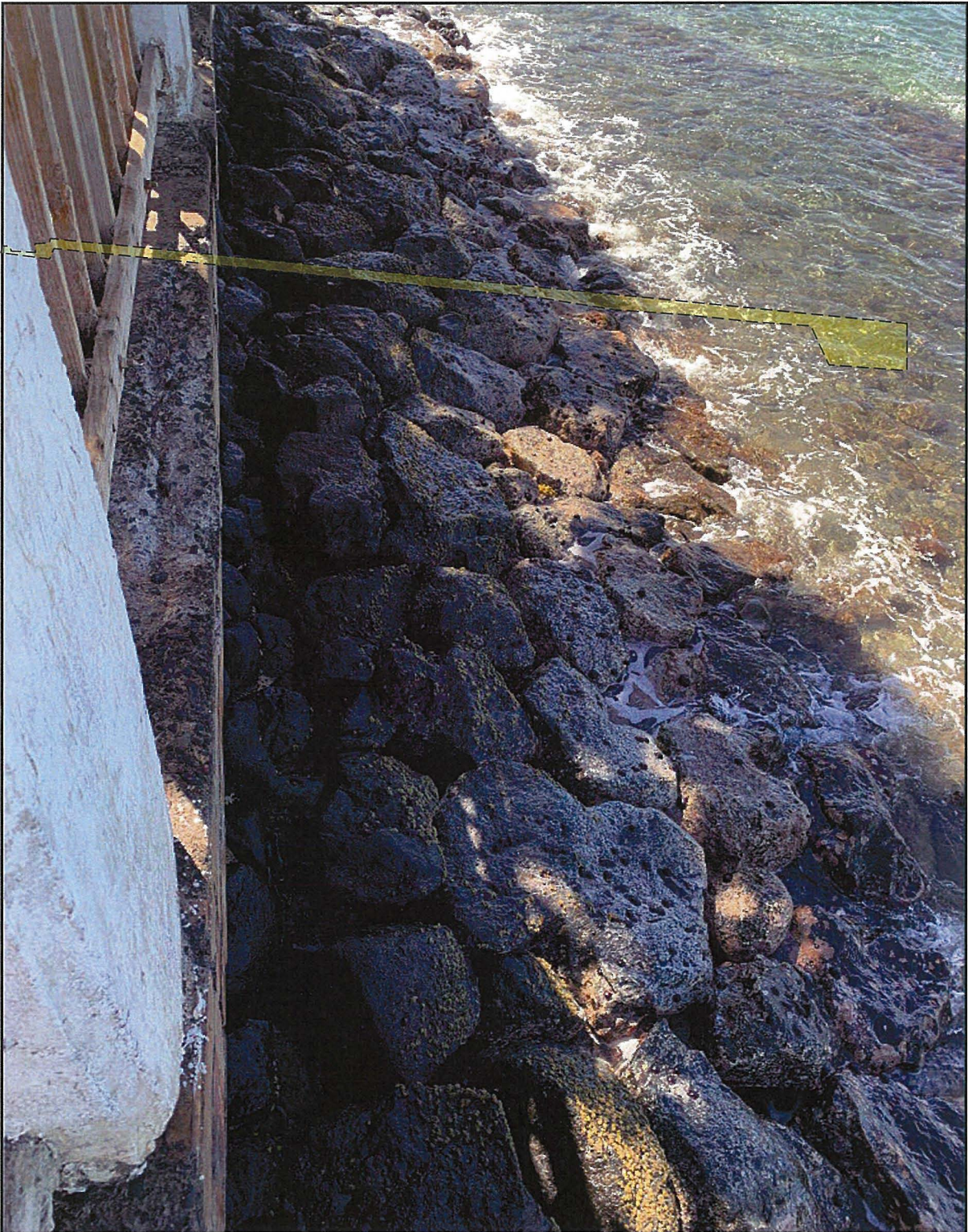
Note: Area 1, revetment (stacked rocks) looking southeast.
