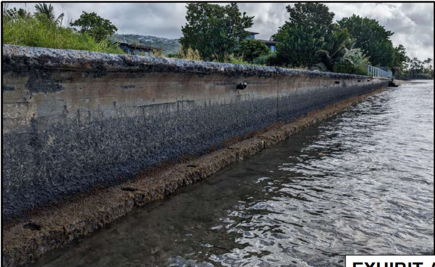
Note: Photo of seawall looking east.
