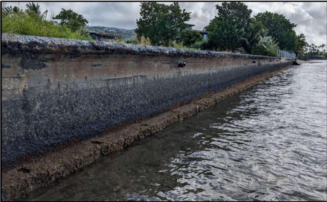
Note: Photo of seawall looking east.
