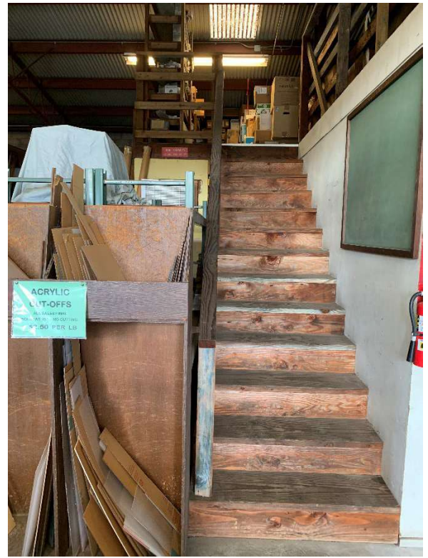
MEZZANINE ACCESS STAIRS
