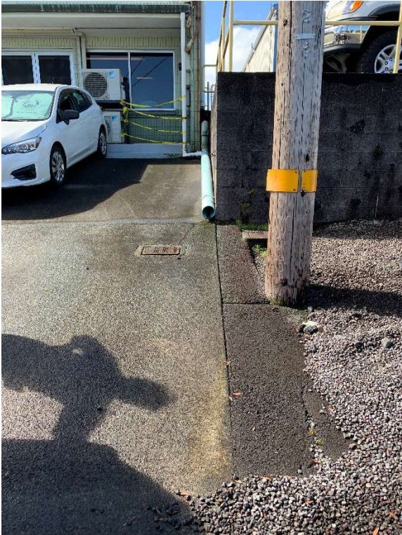
SHARED ROOF DRAINAGE TO STREET
