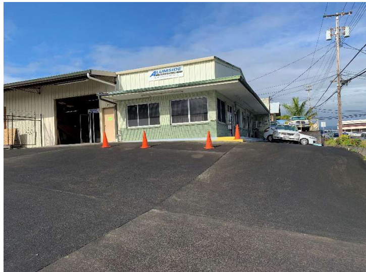
FRONT OF BUILDING FROM STEEP DRIVEWAY. RETAIL, CUSTOMER SERVICE AND OFFICE AREAS IN GREEN PORTION. WAREHOUSE AREA BEGINS AT BAY DOOR.
