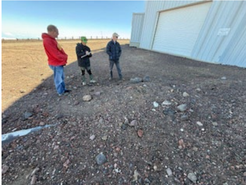
Fig 1. The aboveground conduit transitions to below-ground approximately 30 ft from the north side of the Gemini North Observatory dome.
