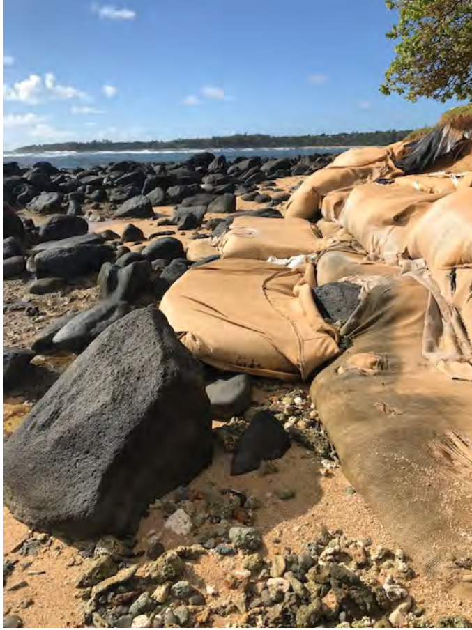
9/3/2020 Photo of Shoreline Area fronting Parcel 004
