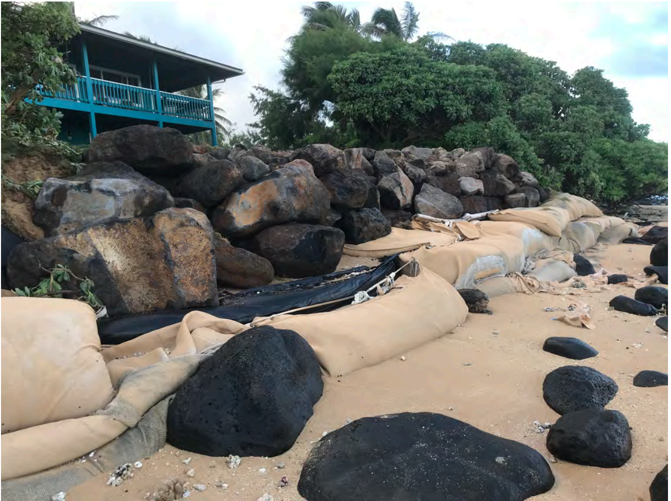
11/16/2020 Photo of Shoreline Area fronting Parcel 004
