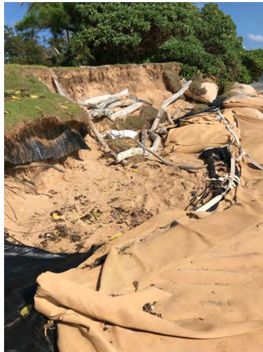
10/7/2020 Photo of Shoreline Area fronting Parcel 004
