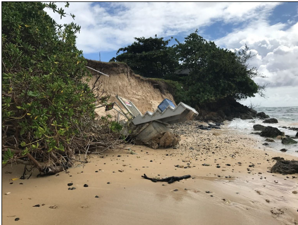
Figure 2-9 Current condition of the shoreline, looking north (7/19/2017)
