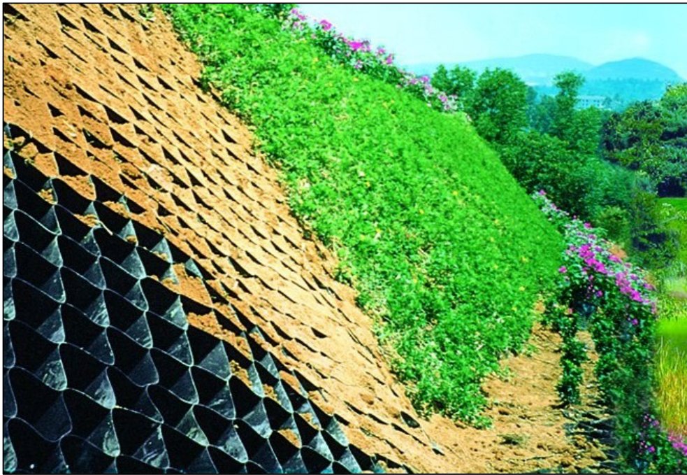
Figure 3-3 Slope stabilization with vegetation and GEOWEB
