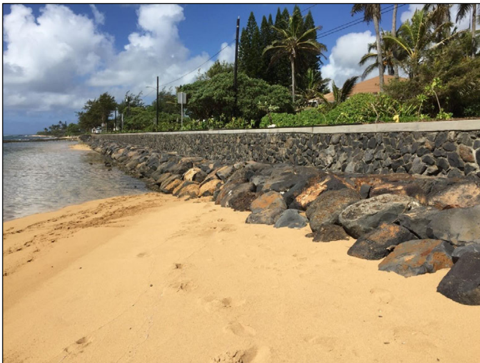
Figure 3-10 Hybrid Seawall-Revetment (Kapaa, Kauai, Hawaii)
