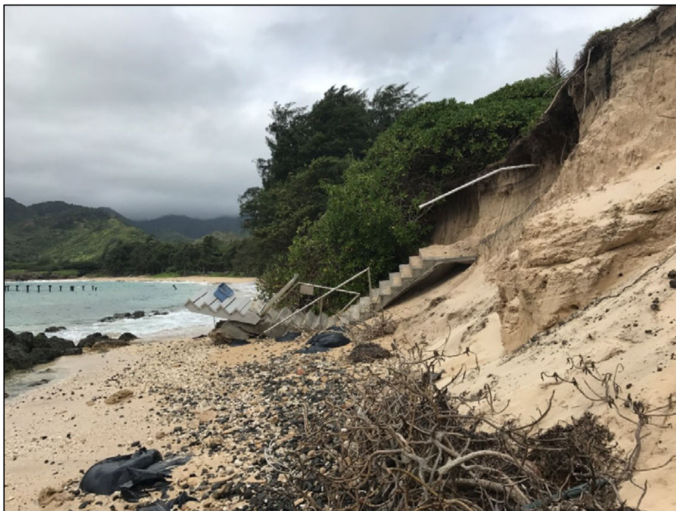
Figure 2-11 Current condition of the shoreline, looking south (7/19/2017)
