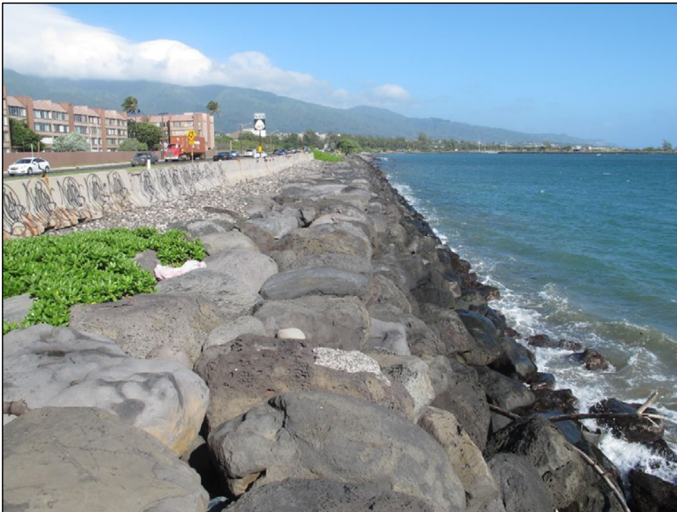
Figure 3-9 Typical rock revetment (Kahului, Maui, Hawaii)
