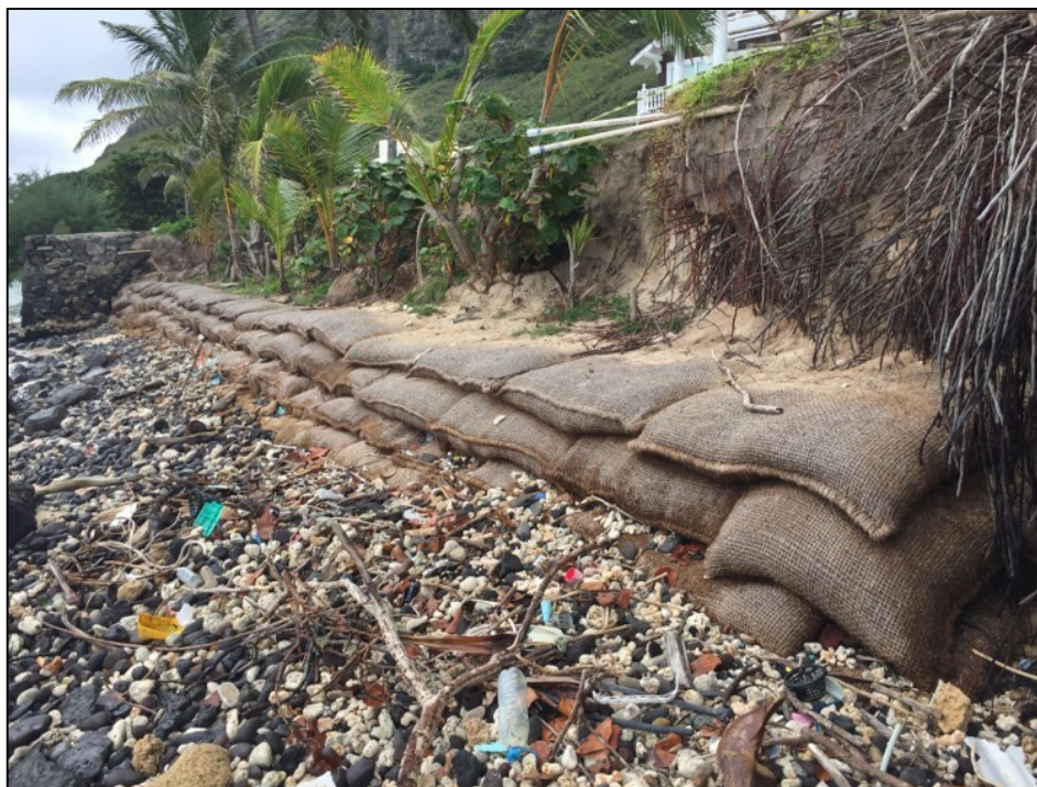
Figure 3-5 Biodegradable sandbag revetment (Waimanalo, Oahu, Hawaii)
