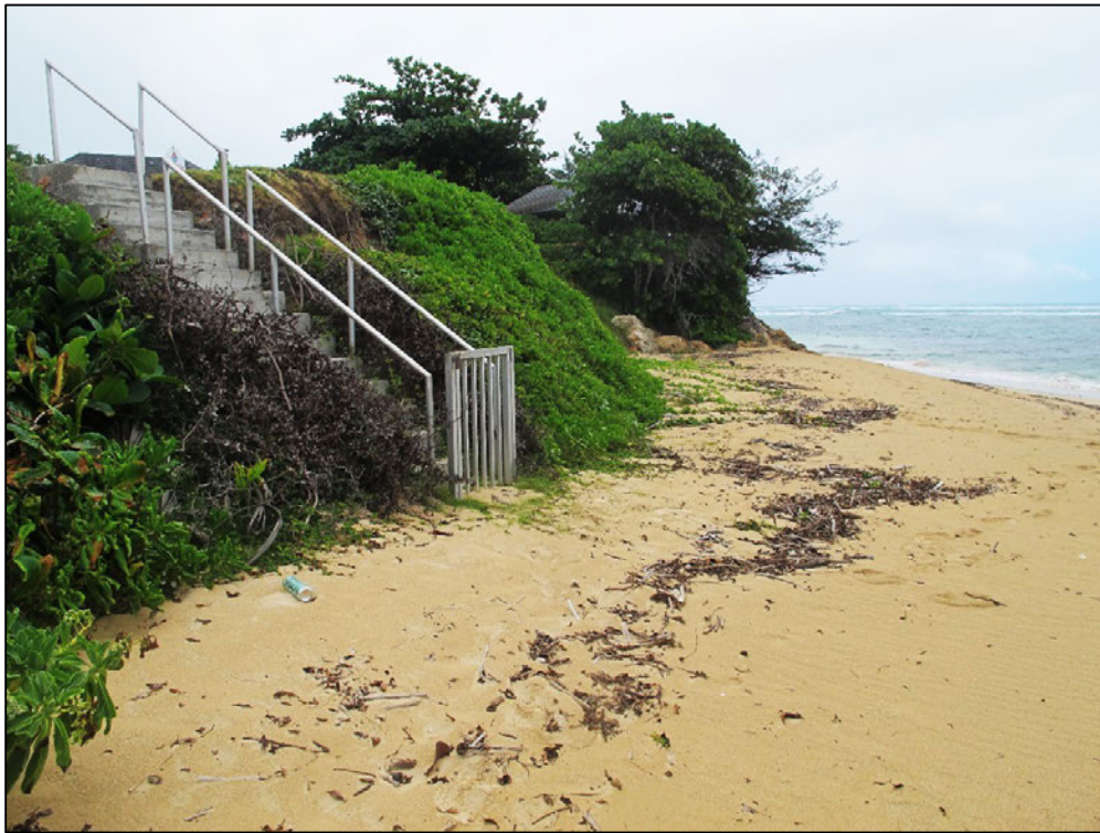
Figure 2-8 Previous condition of the shoreline, looking north (6/13/2013)
