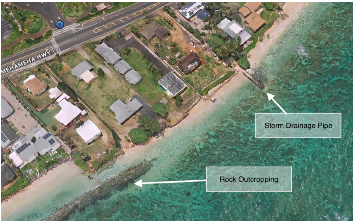
Figure 3-4B: Storm Drainage Pipe
