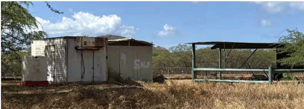
Site inspection photo 2: There are structures for the storage of equipment and feed, and 3 open stable enclosures for horse stabling.
