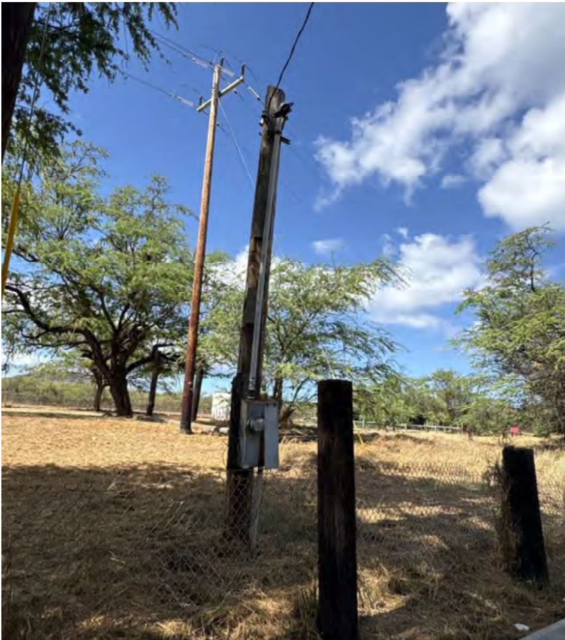
Site inspection photo 4: Easement LOD24350 to Hawaiian Electric Company, Inc.
