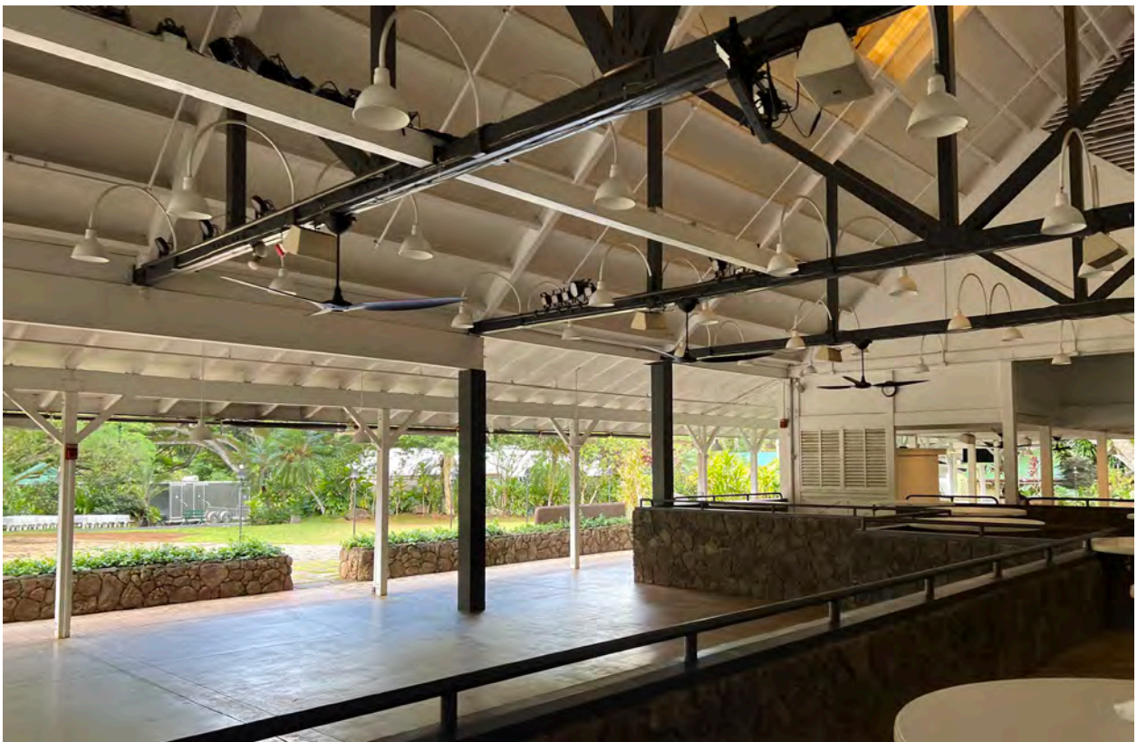
Photo 26. Oblique Interior view of Pikake Pavilion, camera facing west.
