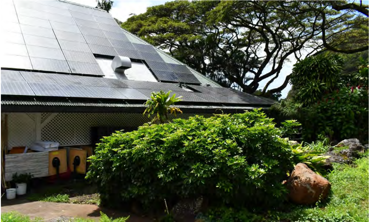
Photo 25. Oblique view of Rear façade of Pikake Pavilion, camera facing northwest.
