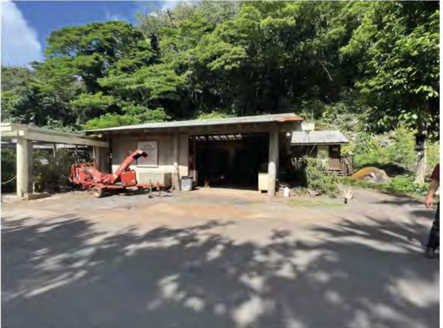
Figure 41. View of Community Resource Center
