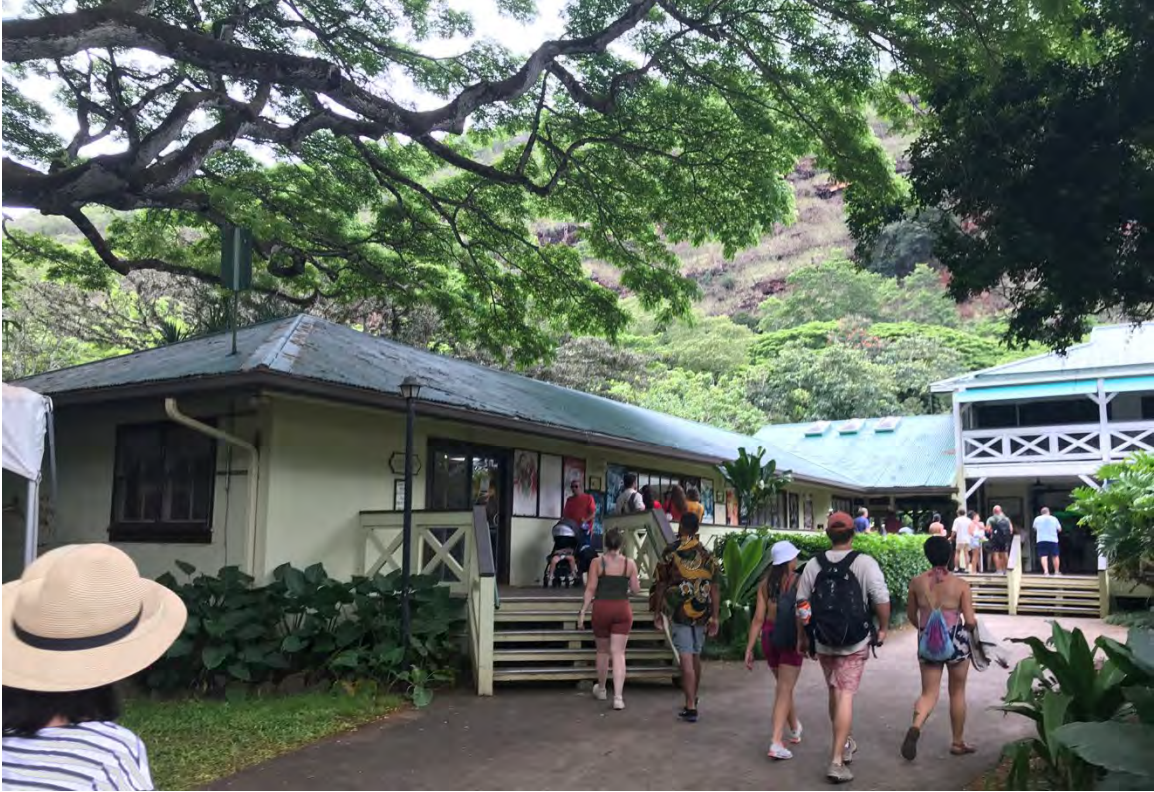
Photo 16. Oblique view of side/rear facades of Gift Shop, camera facing northwest.
