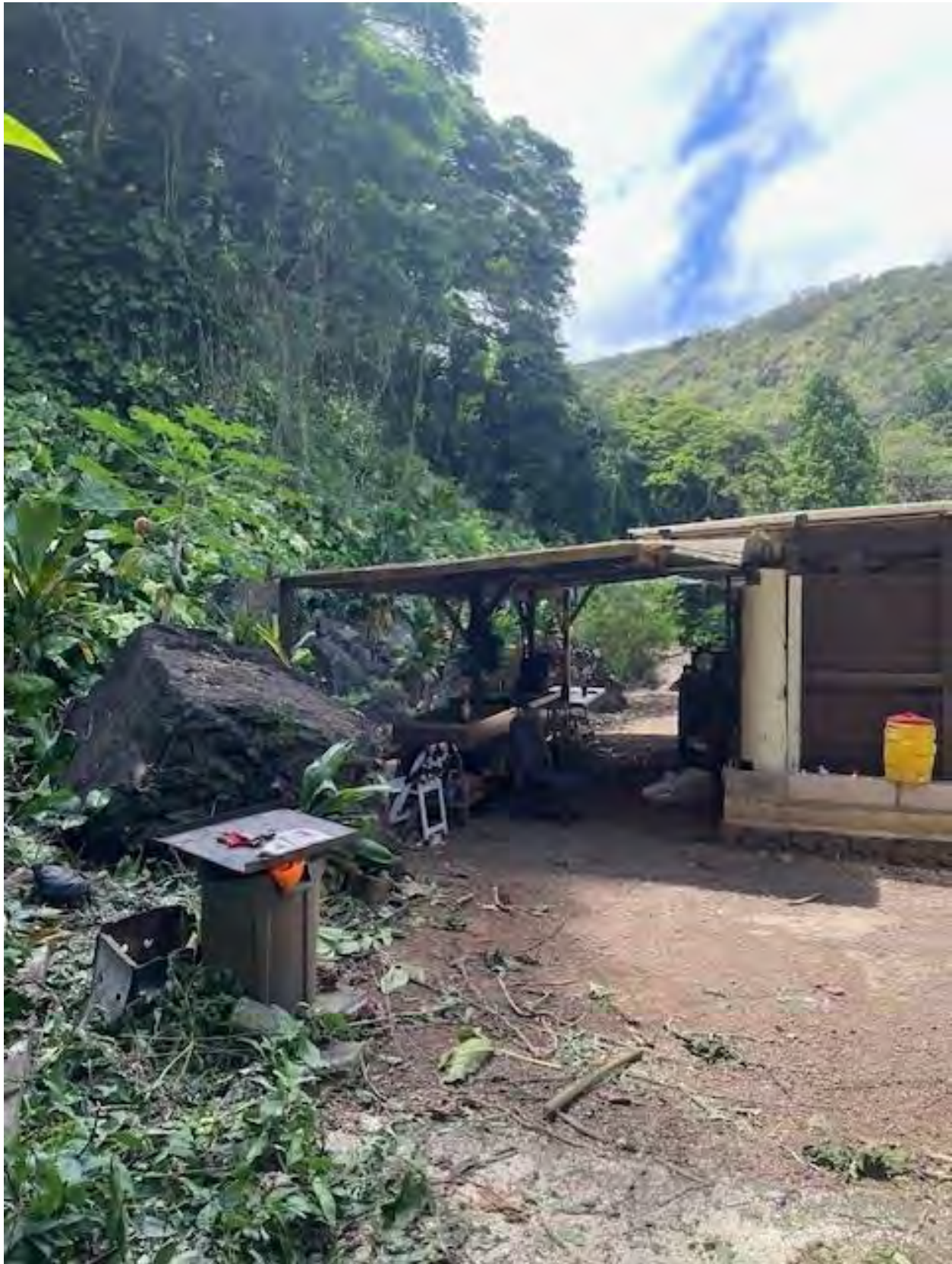
Photo 2. Facing east at the location of the rockfall mitigation behind the Community Resource Center
