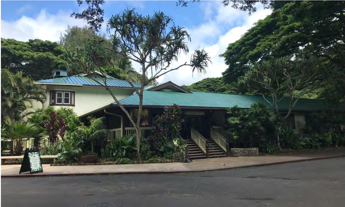
Photo 6. Front façade entry to Visitors Center, camera facing southeast.
