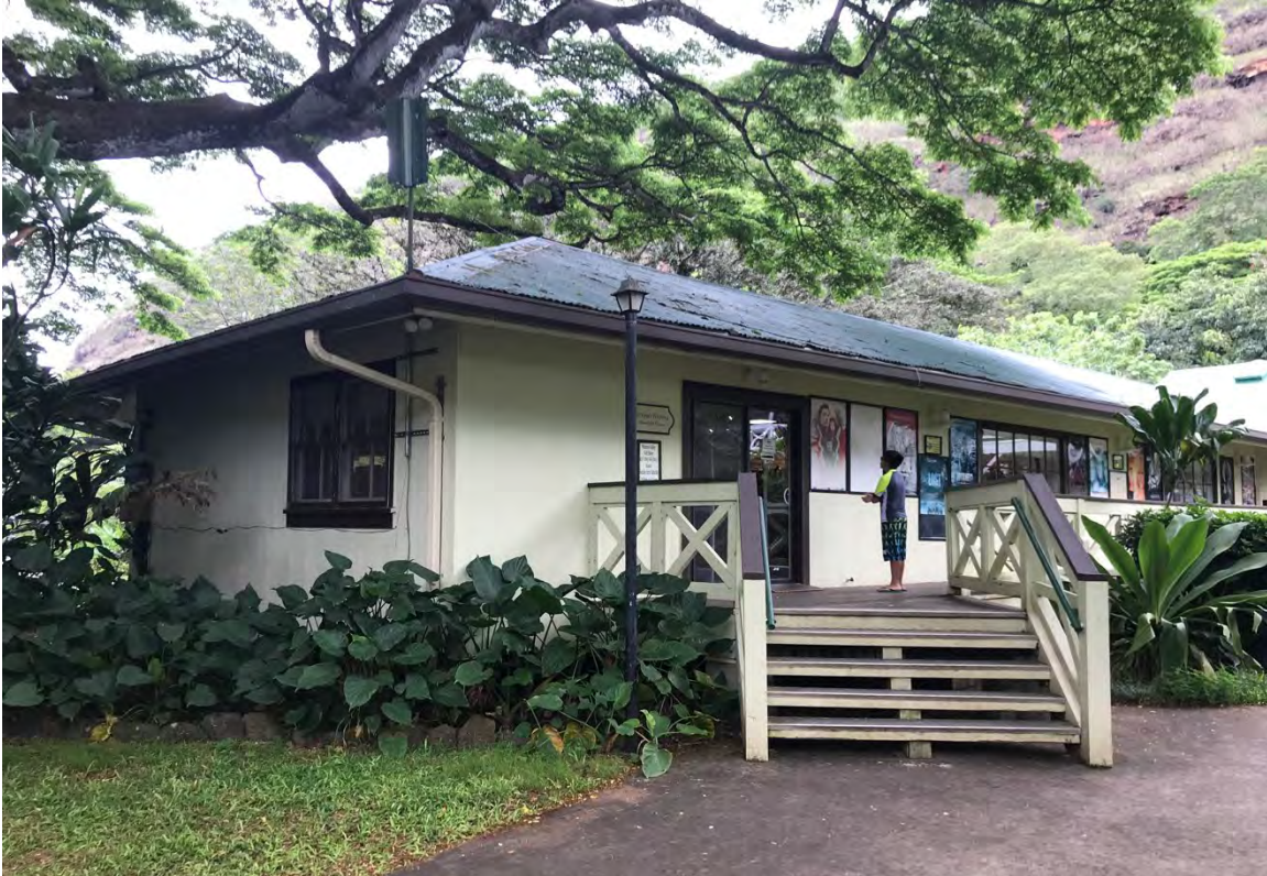
Photo 14. Oblique view of side and rear facades of Gift Shop from courtyard, camera facing northwest.
