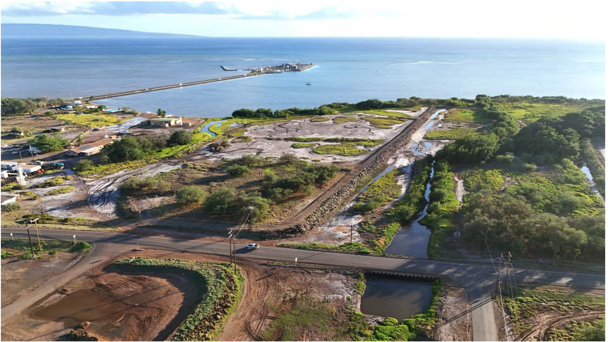
Property fronts Maunaloa Highway, near town core and Kaunakakai Wharf
